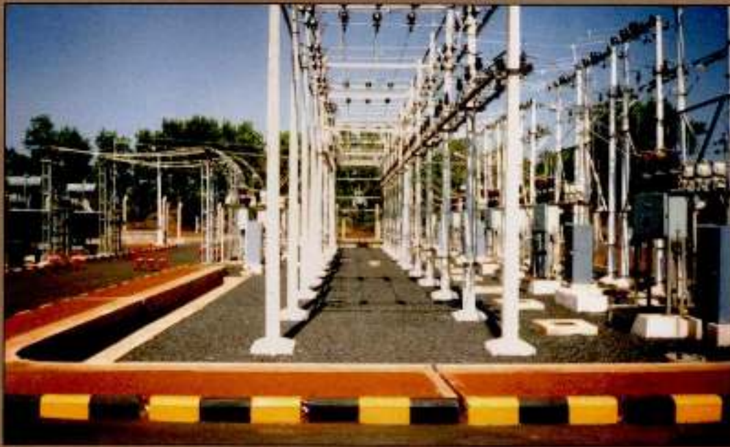
Establishing of 33/11 KV sub station at uchagoan Belgaum District - Karnataka
